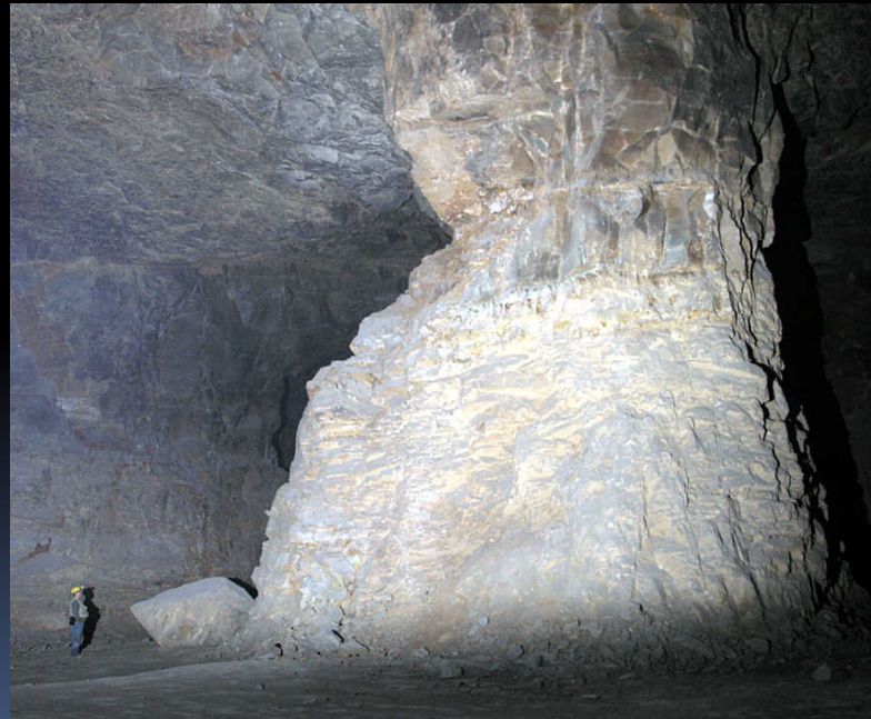
Pillar rib failure in a limestone mine
