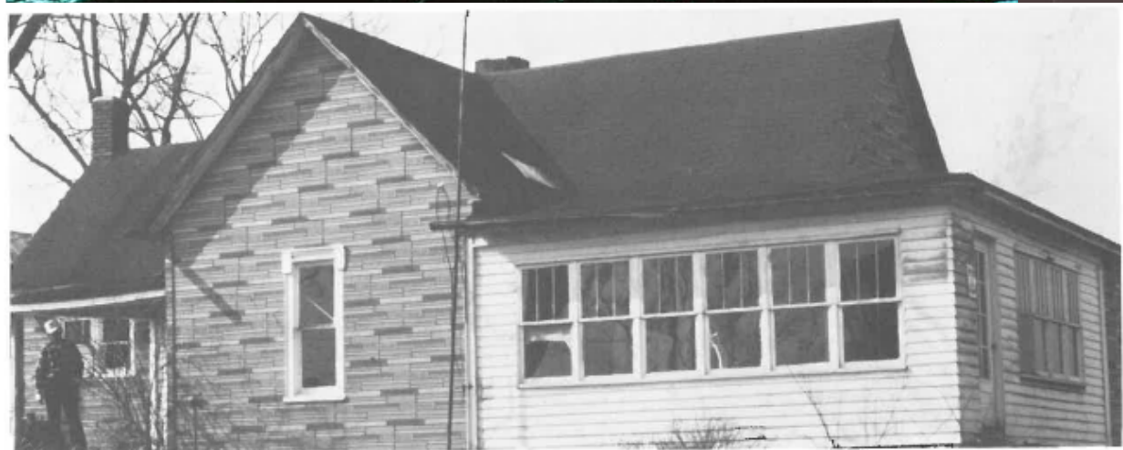
Figure 21.—Test structure 27, near a coal mine.
