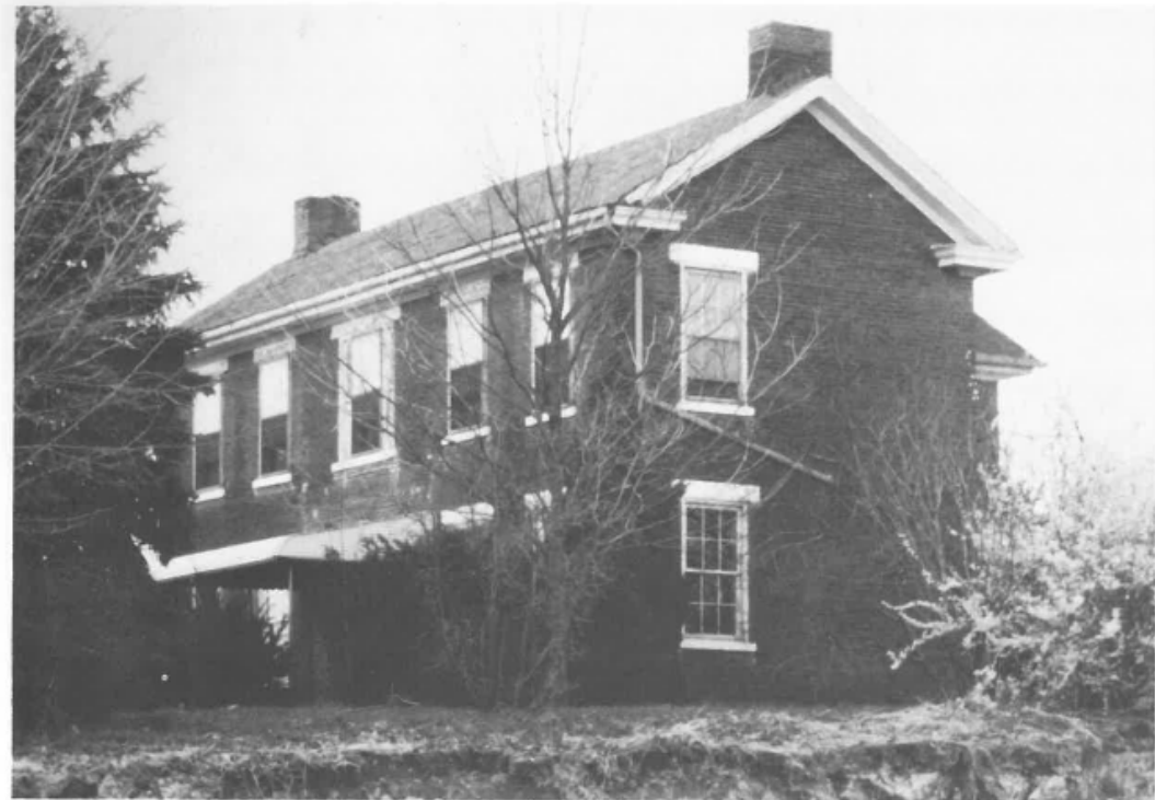
Figure 27.—Test structure 51, near a coal mine.
