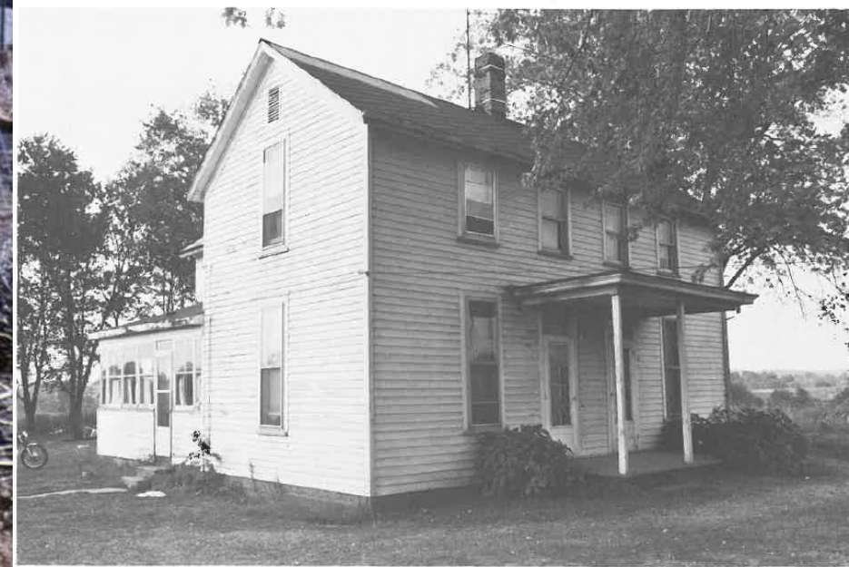
Figure 15.—Test structure 19, near a coal mine.
