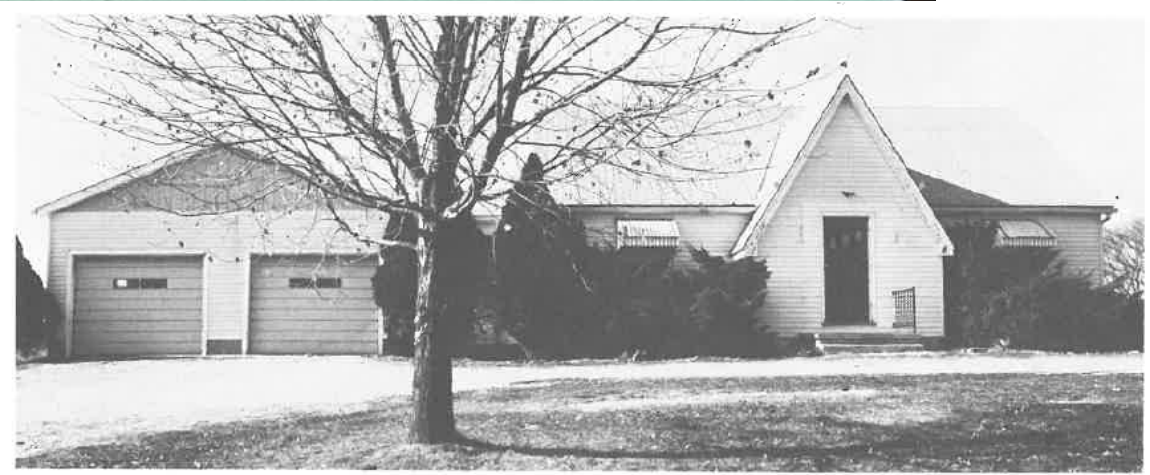
Figure 16.—Test structure 20, near a coal mine.
